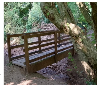
Footbridge over 'Tim Syke'
